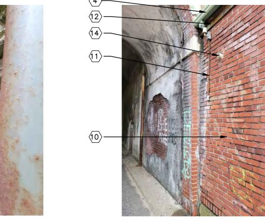
PHOTO 1: BRICK WALL AND CONDUIT AT NORTH WALL OF ELECTRICAL ROOM
